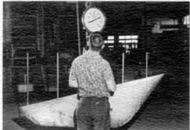
9. All raw lead ballasts are weighed when received from the foundry to insure uniform weight in each keel.
