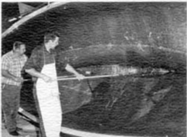
2. The resin is rolled out to avoid air entrapment.
